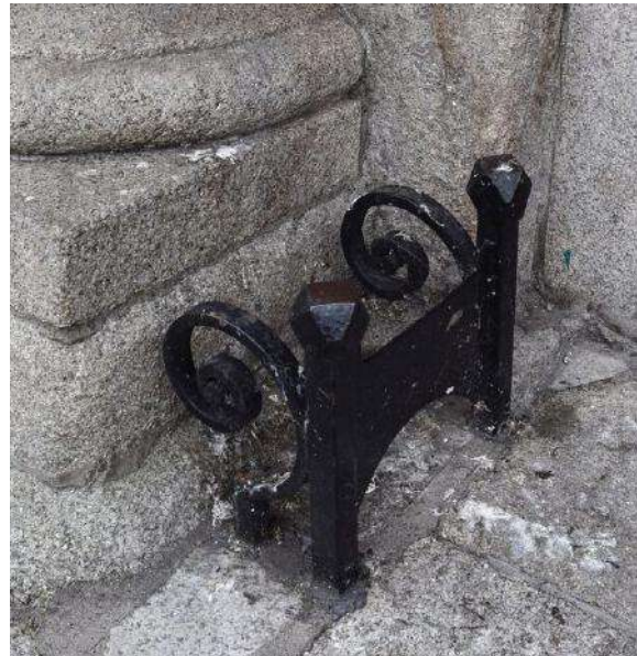
PLATE 28 Cast iron bootscrapes to west and north entrances.
