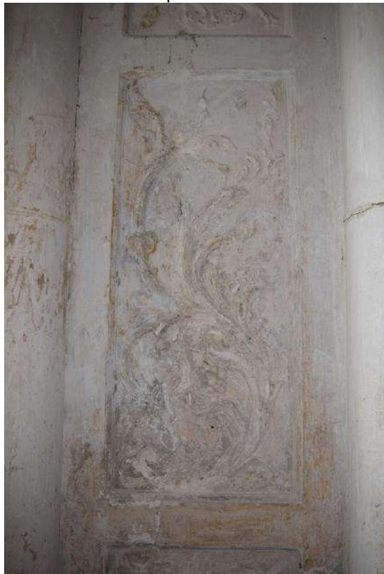
PLATE 37 Detail of plasterwork in Chancel
