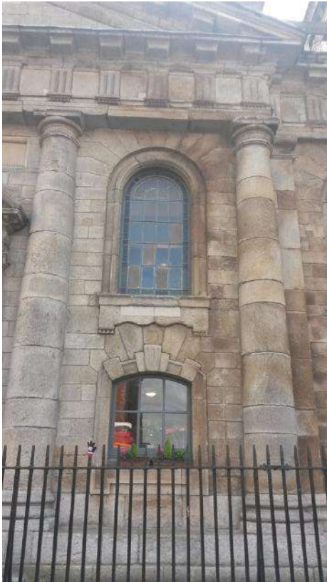
PLATE 5 North façade, Bay 4
