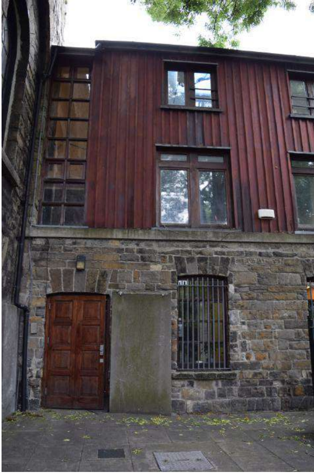
PLATE 14 Contemporary extension to upper levels. Original vestry building at ground level.
