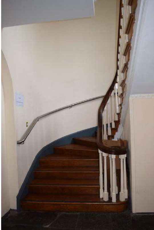
PLATE 38 Refurbished stairs – North west corner of structure
