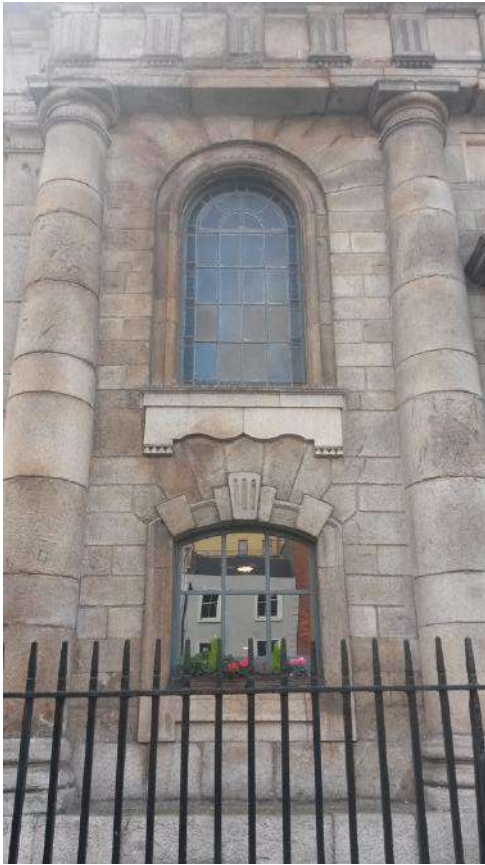
PLATE 3 North façade, Bay 2
