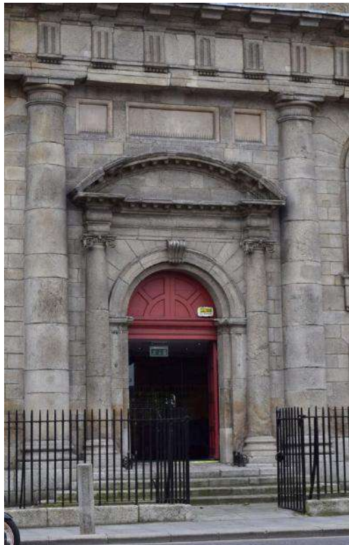
PLATE 4 North façade, Bay 3/ Central Bay
