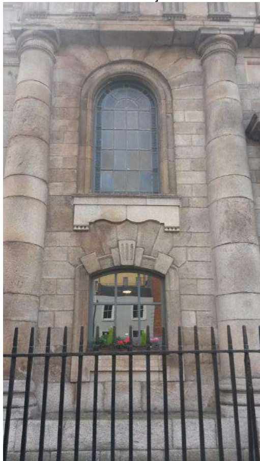
PLATE 2 North façade, Bay 1
