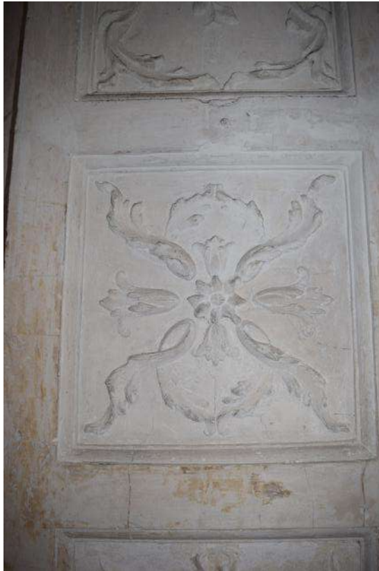
PLATE 36 Detail of plasterwork in Chancel
