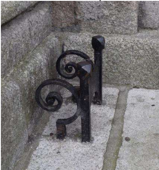
PLATE 28 Cast iron bootscrapes to west and north entrances.
