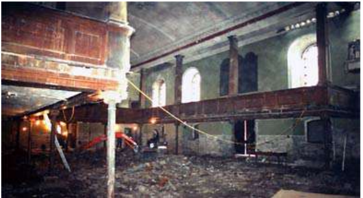
Plate 9 Interior view during restoration works to the interior c1998 above
