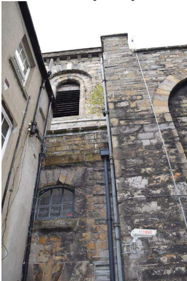
PLATE 17 Junction with adjoining structure on Thomas Court
