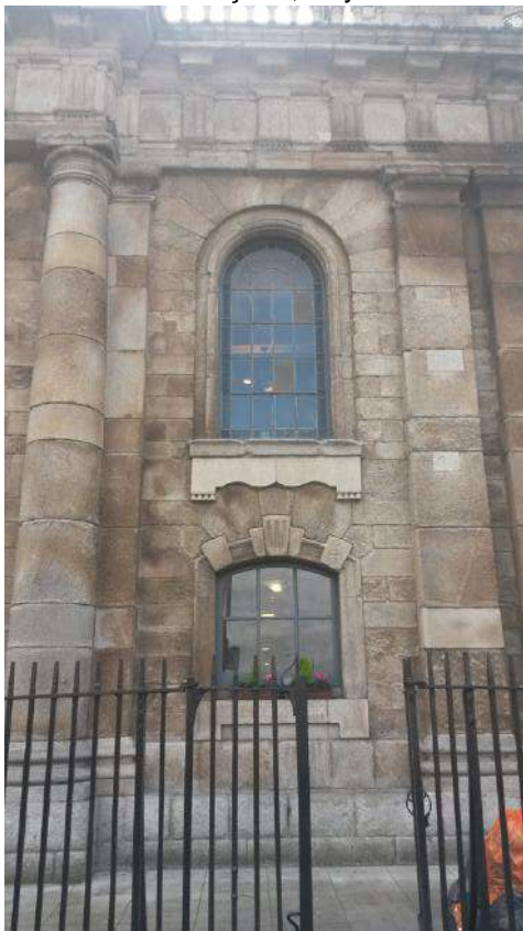
PLATE 6 North façade, Bay 5
