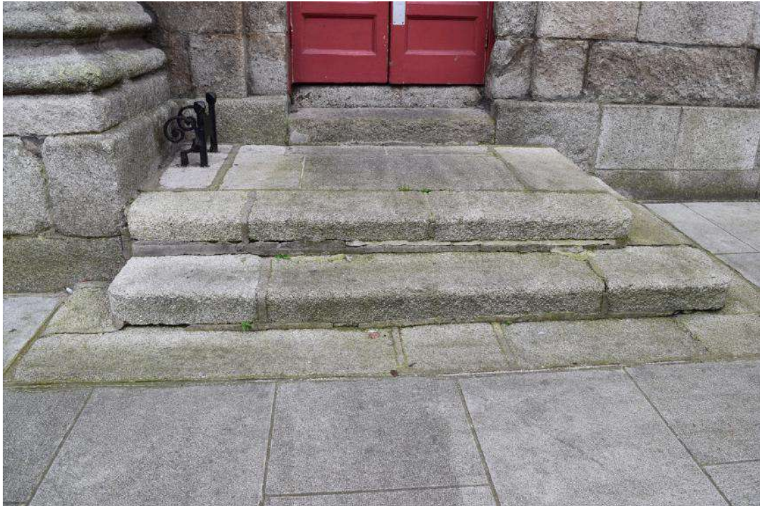
PLATE 11 Granite steps to secondary entrance, North elevation
