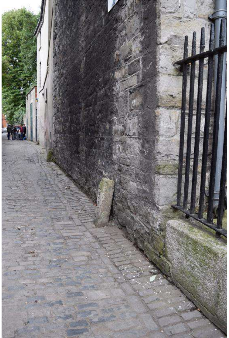
Above: Plate 10, St. Catherine's Lane stone setts and granite guard stones.
